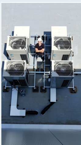
Mooiste foto Martin Hartman CoolCareHolland
